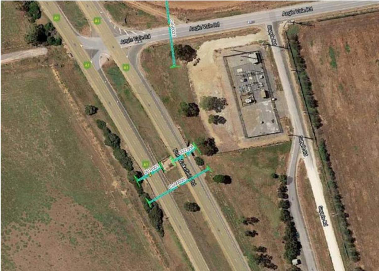
Figure 10: Port Wakefield Road Culverts
