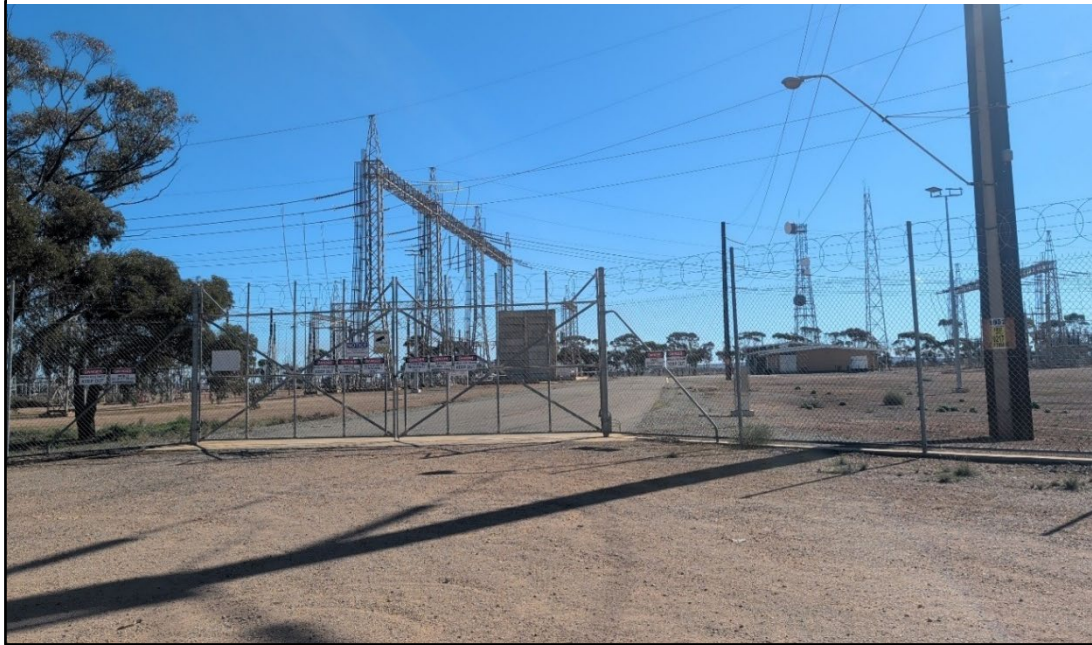
Figure 5 - View along Power Station Road into the existing Brinkworth Substation
