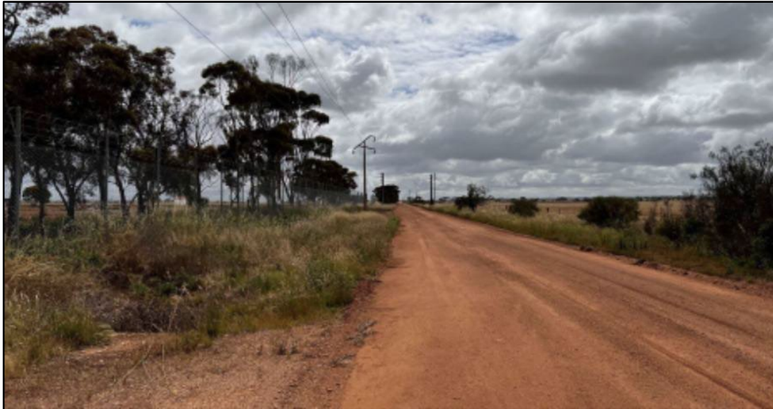
Figure 6 - View along Power Station Road where the underground transmission cable will be located on the right-hand side of the image. The Brinkworth Substation is located on the left-hand side of the image
